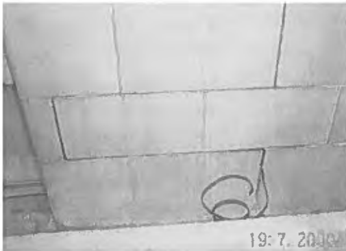
Photograph 2: Ribbon anodes in ashlar jointing
