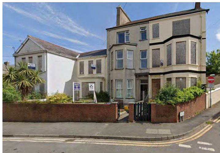
Figure 50 – Dwellings at corner of Southwell Road and King Street
