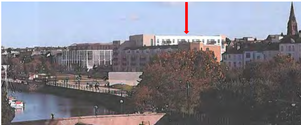
Figure 61 – CGI image of original submission showing additional floor on apartment block facing Market Place.
