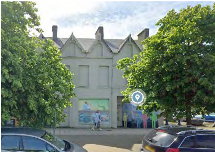
Figure 56 – Existing Buildings at 9-12 Queen's Parade
