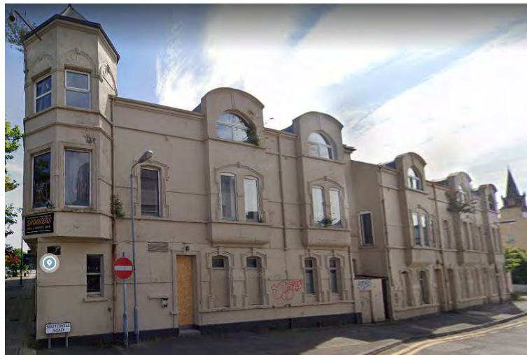
Figure 51 – Building at corner of Southwell Rd and Queen's Parade
