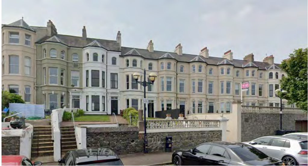
Figure 24 – Existing residential terraces on Queen’s Parade
