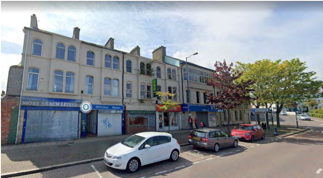
Figure 55 – Existing Buildings at 35-41 Queen's Parade Proposed for Demolition
