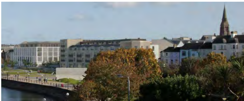
Figure 62 – CGI image showing amended scheme with top floor facing Market Place removed and replaced with additional floor fronting Queen's Parade
