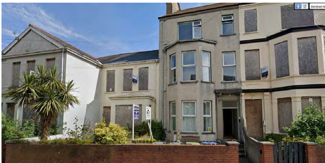
Figure 82 – Existing buildings on Southwell Road
