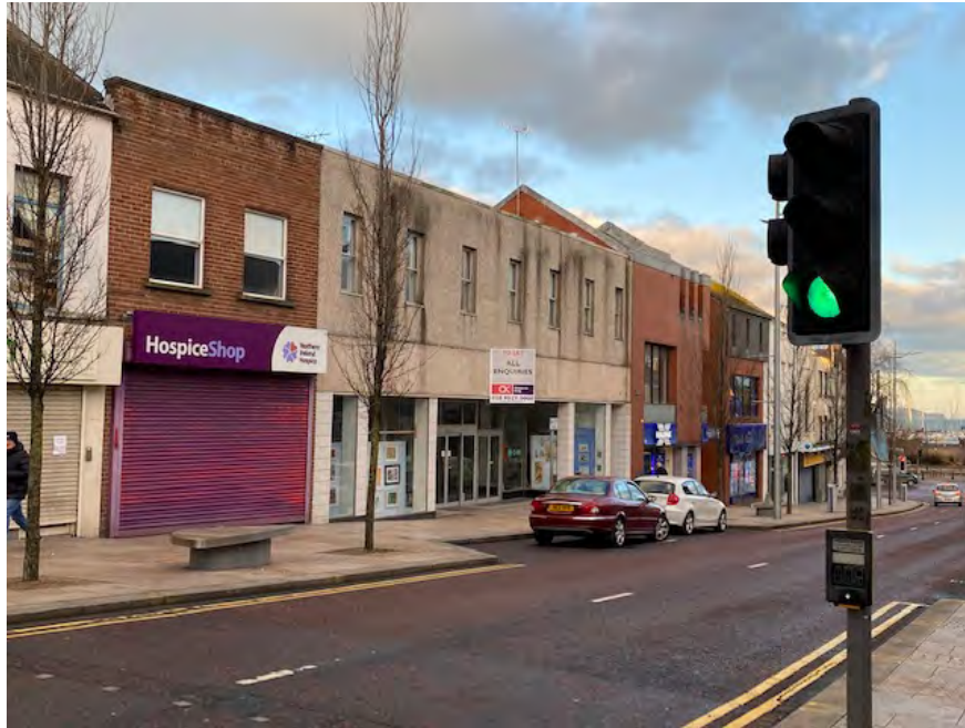
Figure 39 – Existing buildings on Main Street to be demolished
