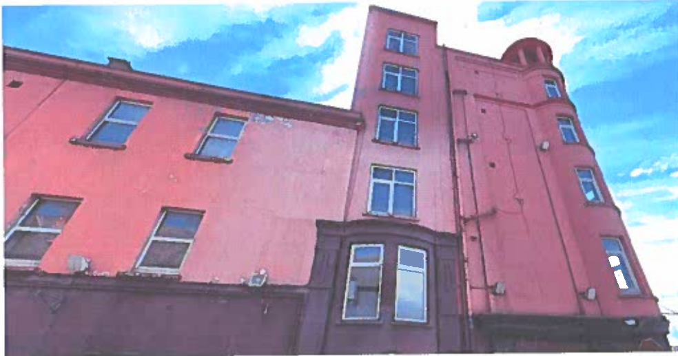
Plate 2. Site of former Royal Hotel from corner with Crosby Street.
